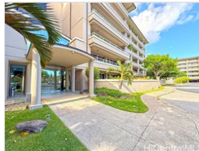
Building Two Entry
